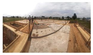
The forms for pouring the concrete roof for the first level which is the floor for second level of the building are completed.
